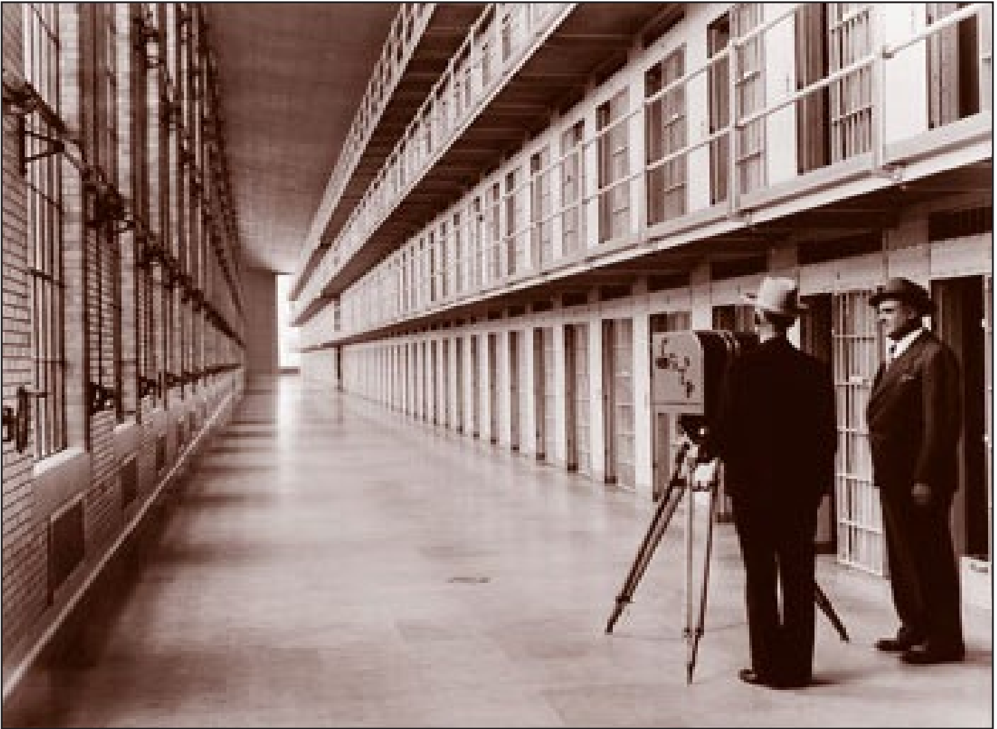
Warden and deputy warden demonstrating possible use of television cameras for security purposes at the State Prison in 1939
