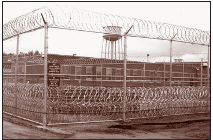
Conversion of the Moose Lake Regional Treatment Center to the Moose Lake Correctional Facility was completed in 1997
